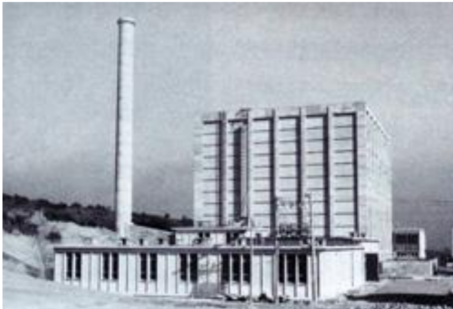
Fig. 1. THOR is the first nuclear reactor in Asia. THOR is a 2 MW, light water moderated and cooled reactor of the TRIGA conversion type. License renewed in 2011.
